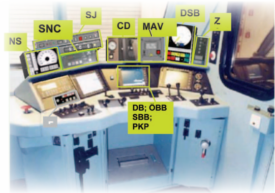
Example of a driver's cab in an international locomotive, where multiple legacy systems are used
